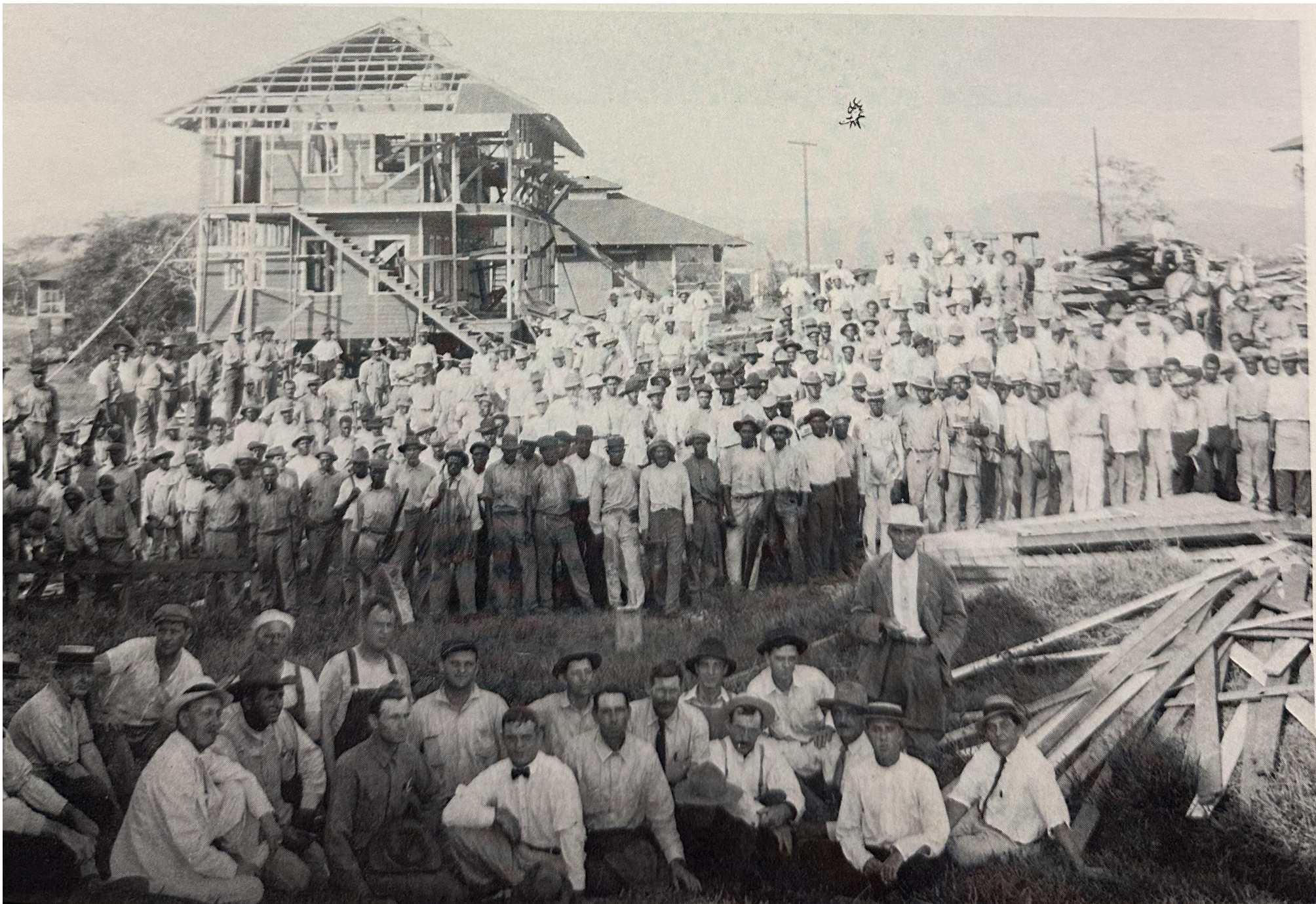
Construction forces re-erecting houses removed from areas to be flooded, Corozal, April 1913. Characteristically, black and white laborers pose in two strictly segregated groups.
