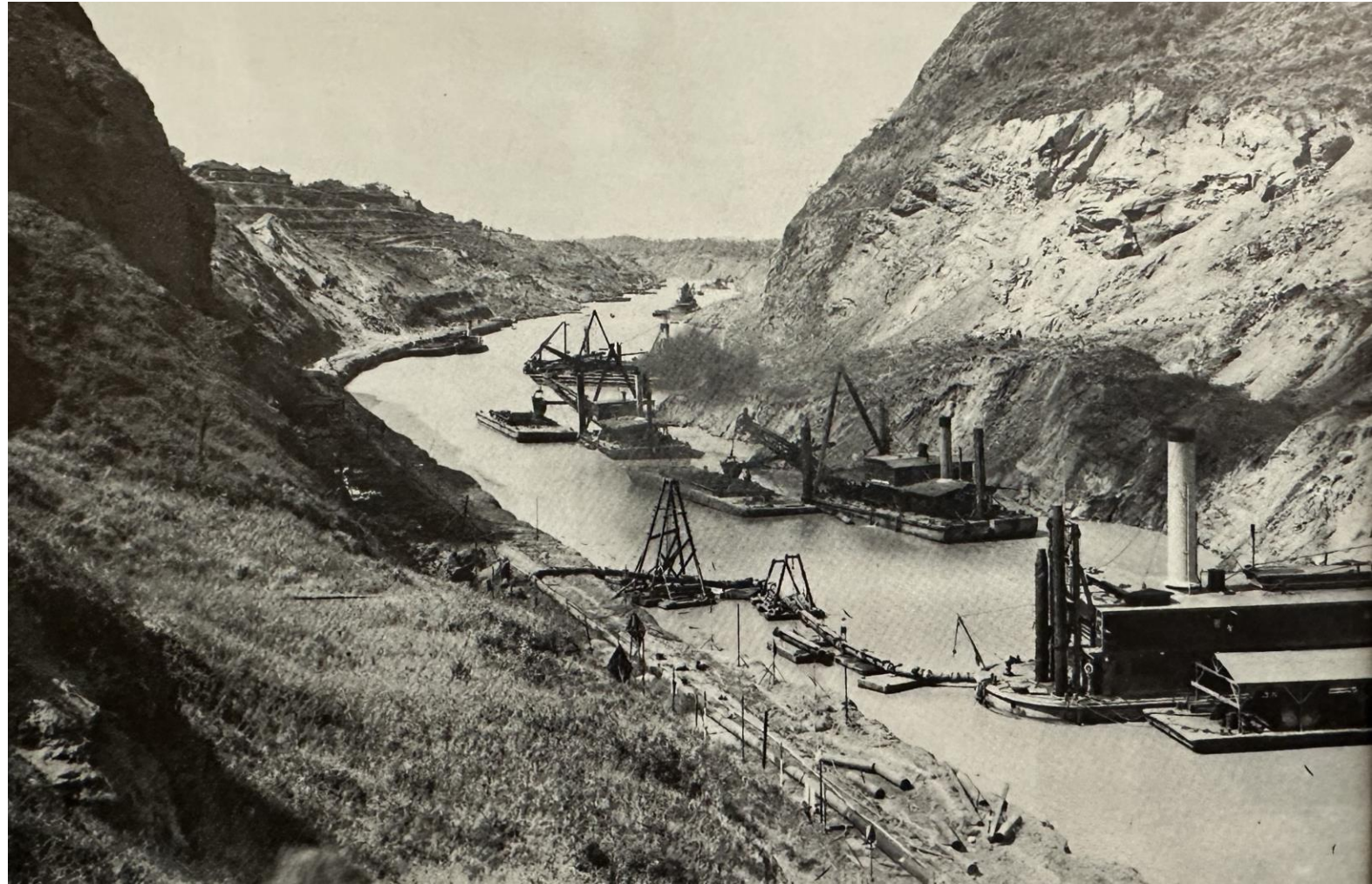
Dredges at work in the Culebra Cut, January 28, 1914.
